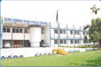
Main Branch GGPS Sector-V, Bokaro
